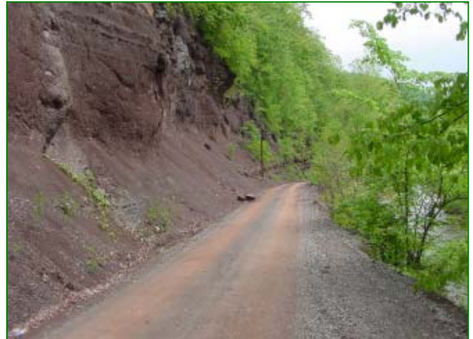
Red silt high-wall along Elk River.
